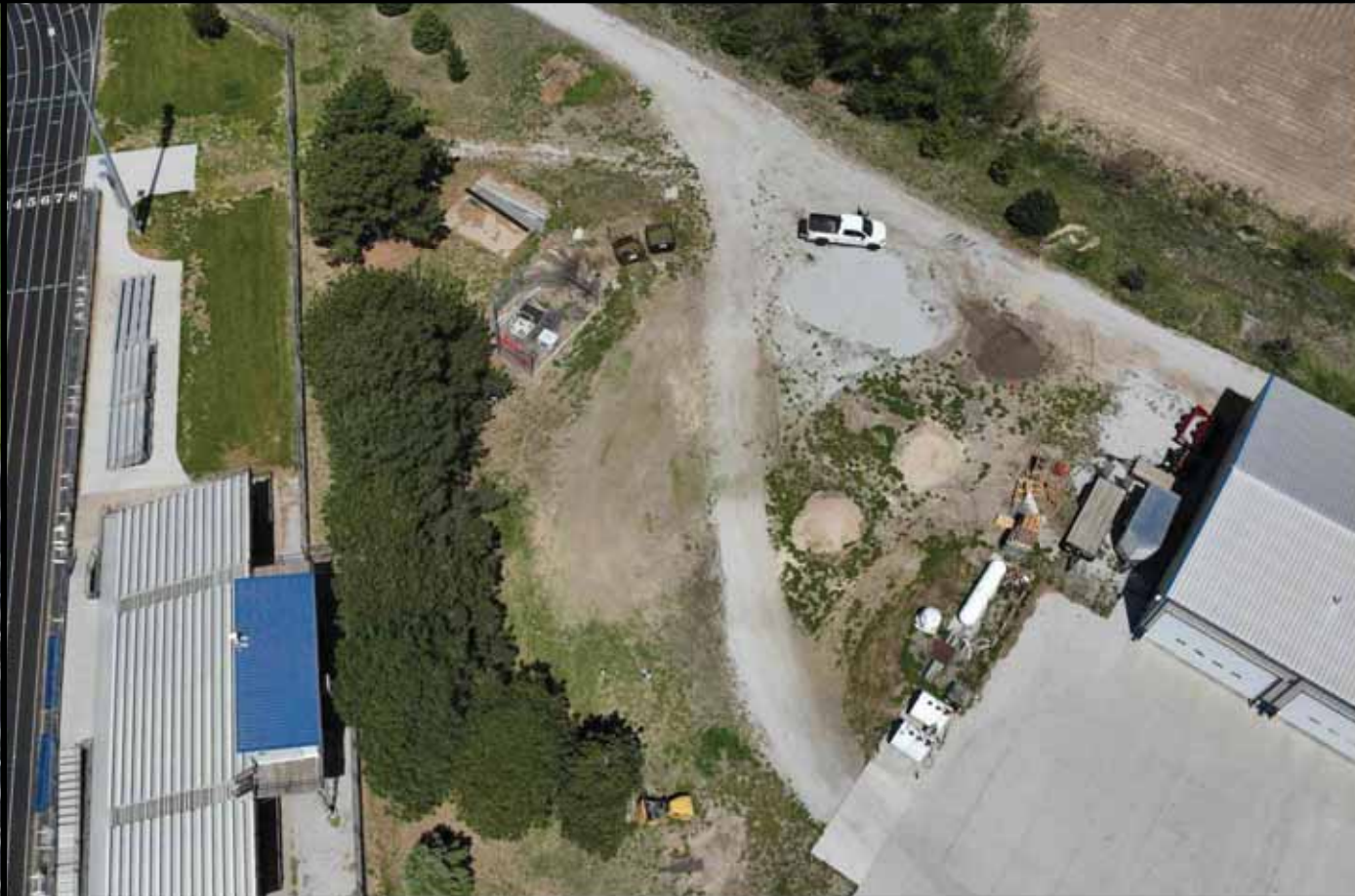
D SITE OVERVIEW (LOOKING NORTHWEST)
