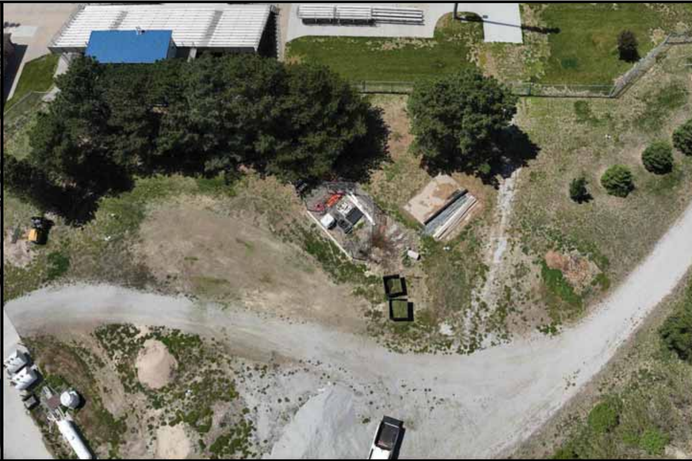
B SITE OVERVIEW (LOOKING SOUTHWEST)
