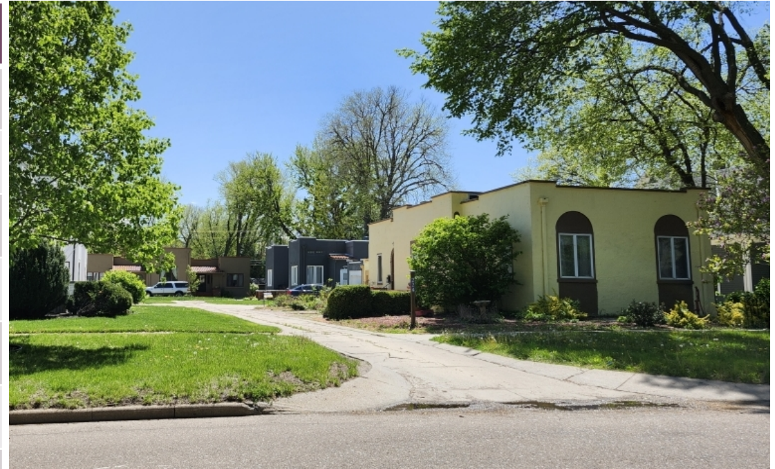
5 units w/ 6 garages
