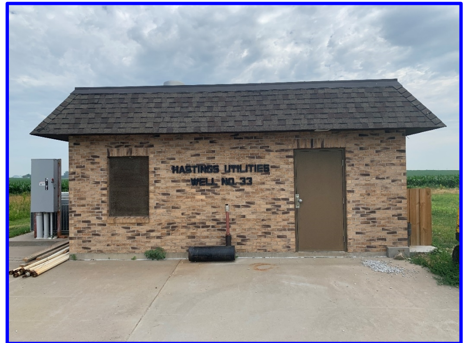
Well 33 Shut Down due to Nitrates
