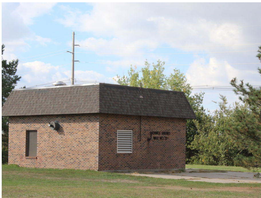
Photo 10.1: Well in operation Source: Marvin Planning Consultants
