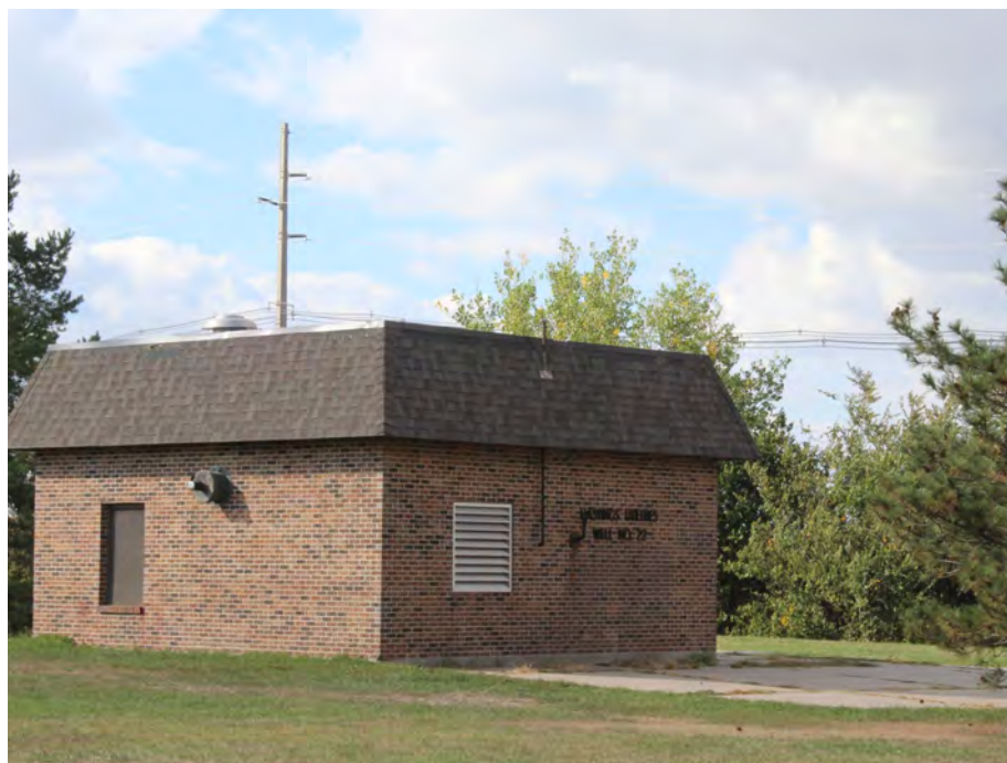
Photo 10.1: Well in operation Source: Marvin Planning Consultants
