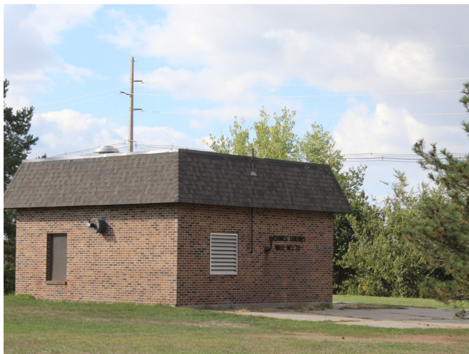
Photo 10.1: Well in operation Source: Marvin Planning Consultants
