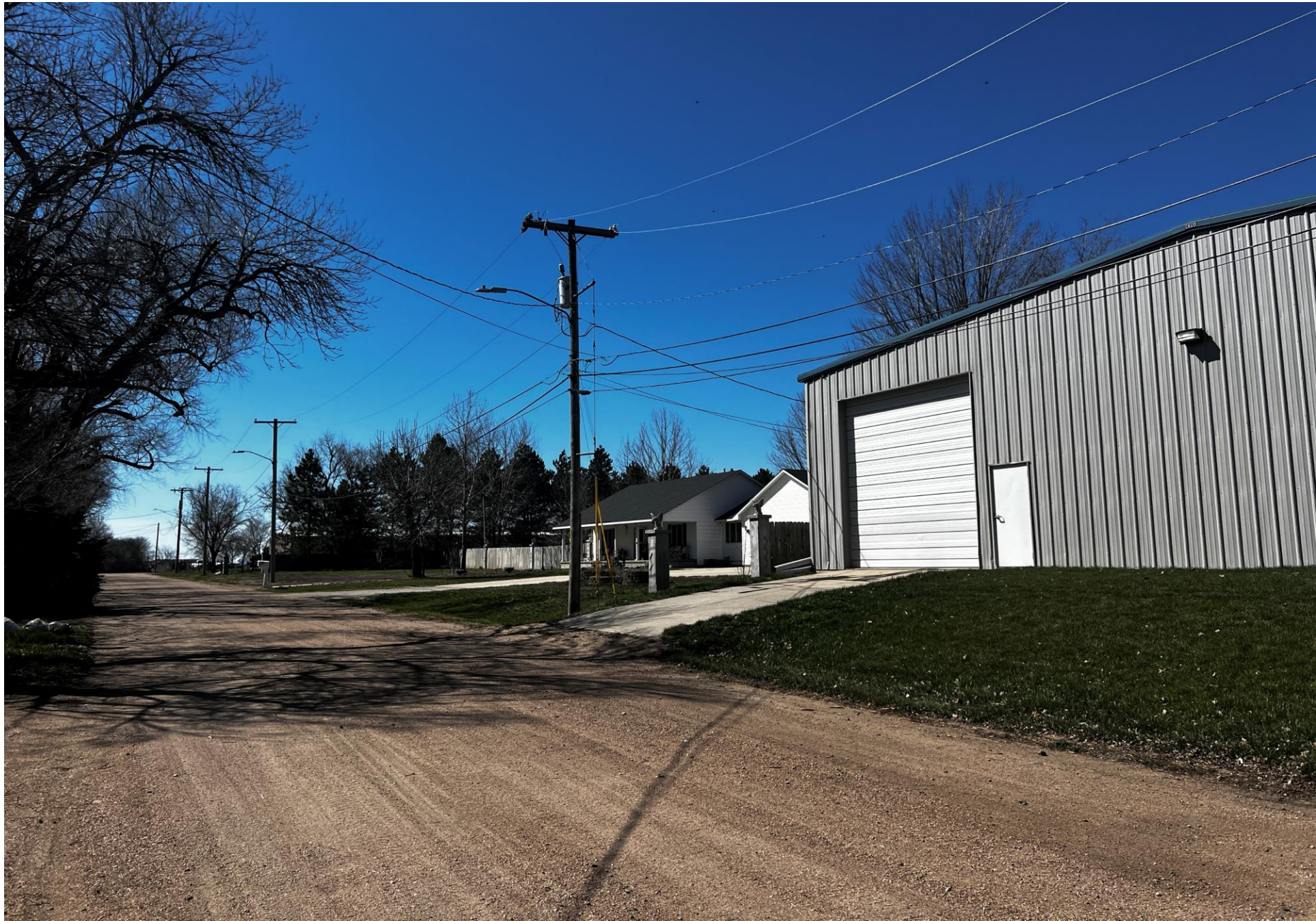
Looking South – Down Cedar Ave.
