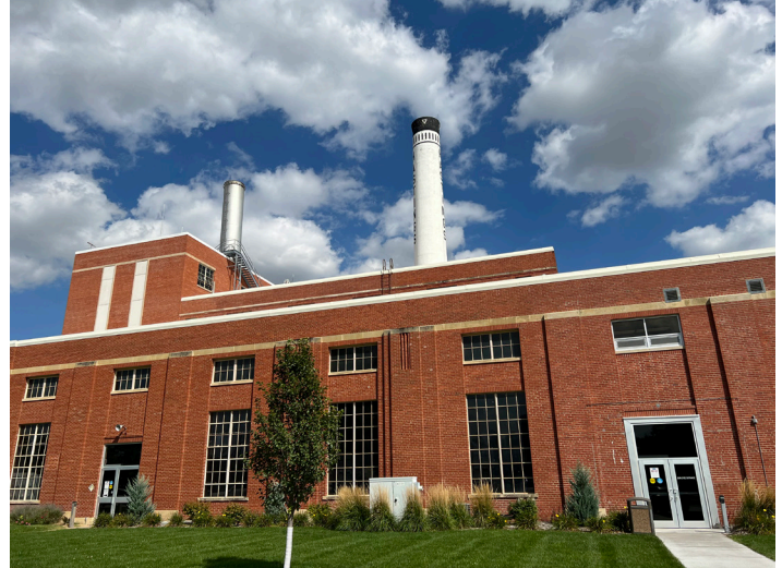
North Denver Station is home to Units 4 and 5, which were repeatedly called into action over the summer, which helps spread some of the fixed cost over more generation, which is a benefit to rate payers.
