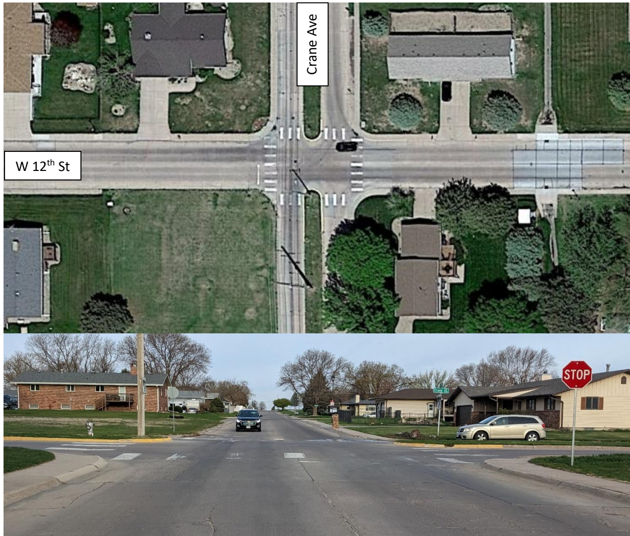
Figure A25: Intersection of W 14 th Street & Crane Avenue (Overhead and Looking West) (Courtesy: Google Earth)
