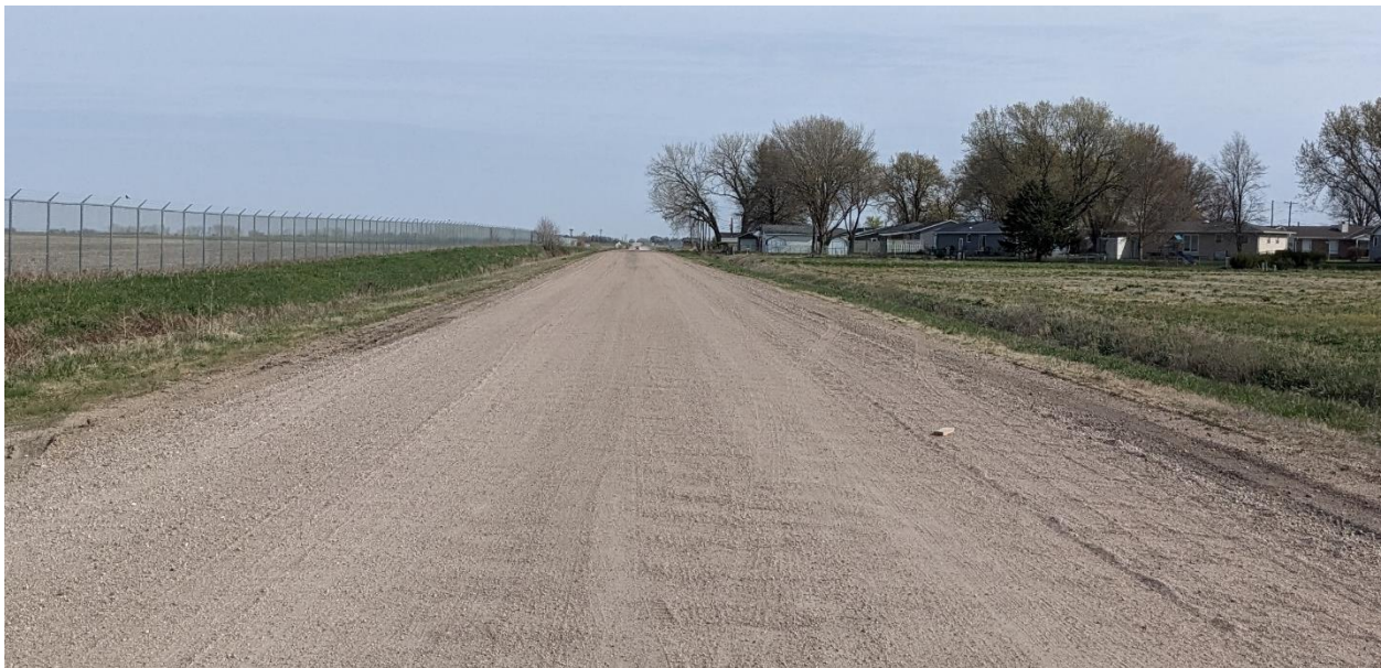
Figure A10: N Marian Road Looking North, North of W 12 th Street
