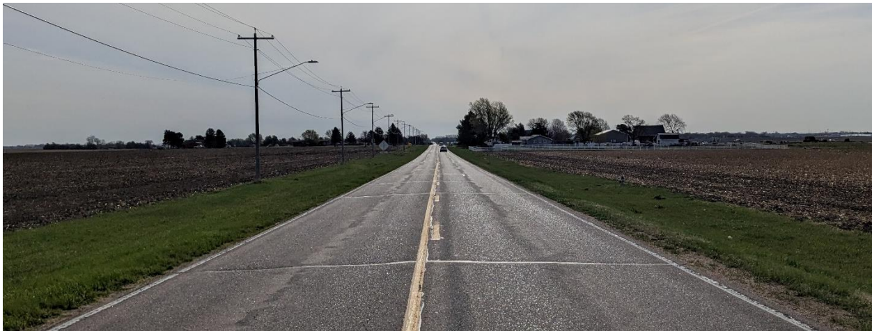
Figure A1: W 12 th Street Looking East, East of N Adams Central Avenue
