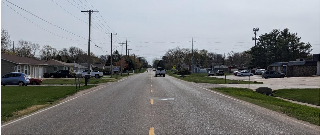
Figure A4: W 12 th Street Looking East, East of N Laird Avenue
