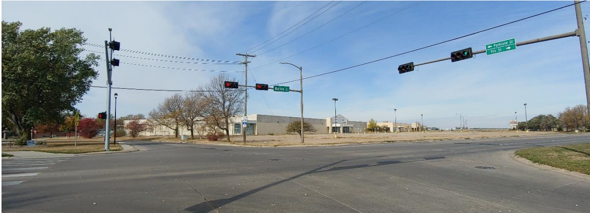
Figure 6: The Intersection of N Marian Road and Parklane Drive/W 9 th Street (Looking Northwest)
