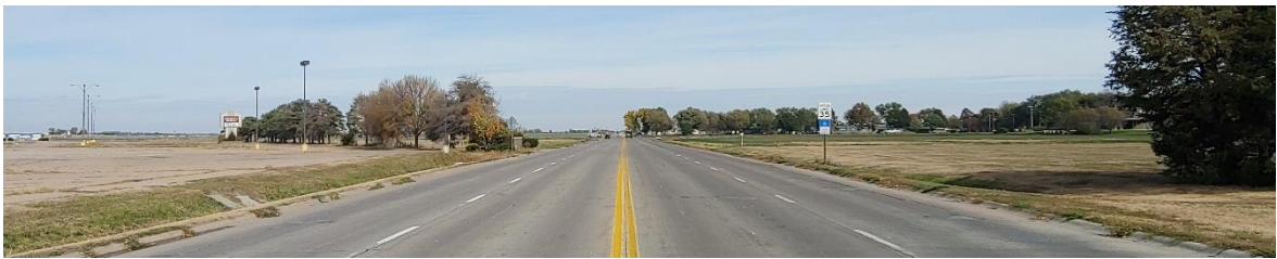
Figure 2: N Marian Road Just North of W 9 th Street (Looking North)
