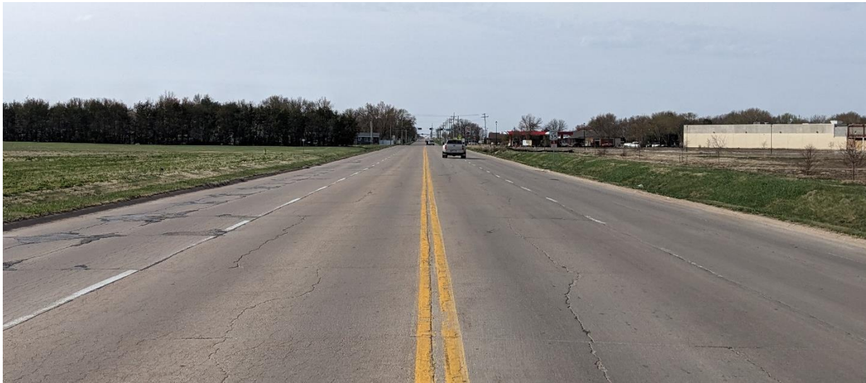
Figure A9: N Marian Road Looking South, South of W 12 th Street
