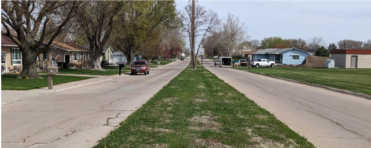
Figure A13: Crane Avenue Looking North, North of W 12 th Street
