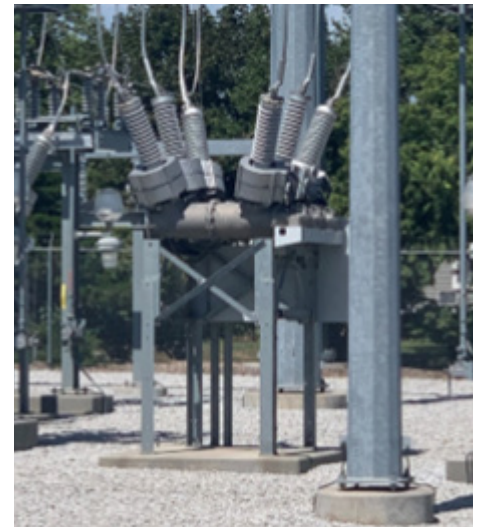
Typical SF6 Circuit Breaker
