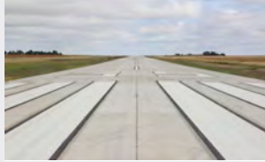
ALLEN COUNTY AIRPORT Iola, KS
