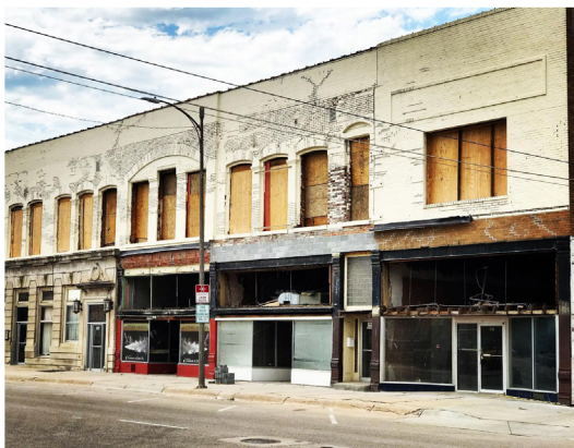
The Cameron Downtown (105 N Hastings Ave.) project came to completion and created 11 studio and one bedroom apartments and 6 retail and commercial storefronts.
