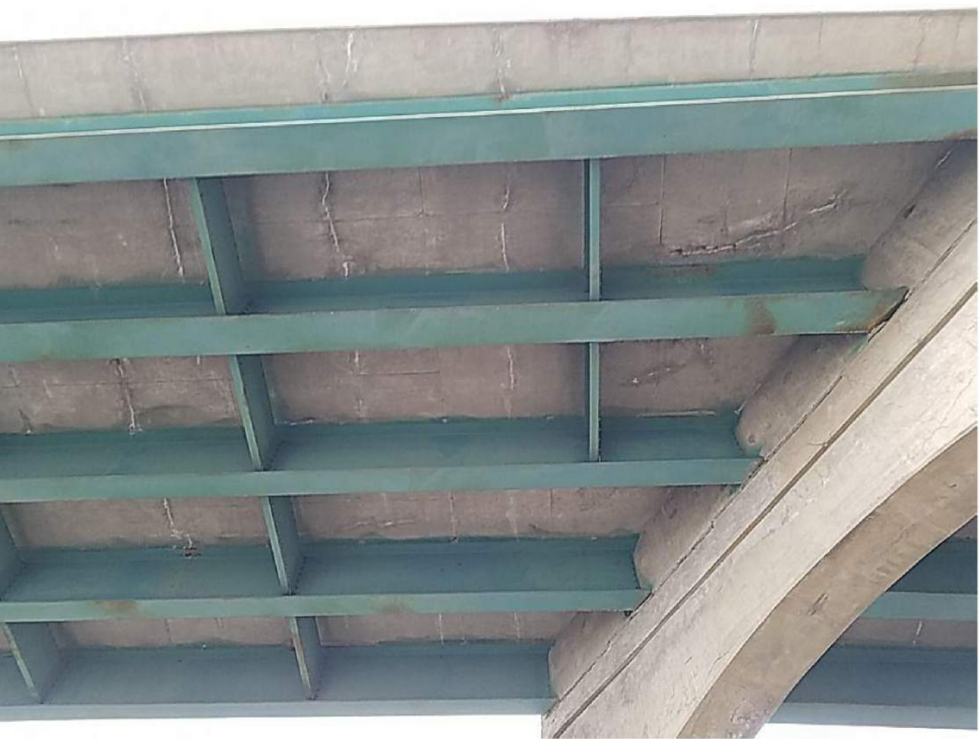
PHOTO 12 - TYPICAL SUPERSTRUCTURE SHOWN AT A FIXED BEARING END
