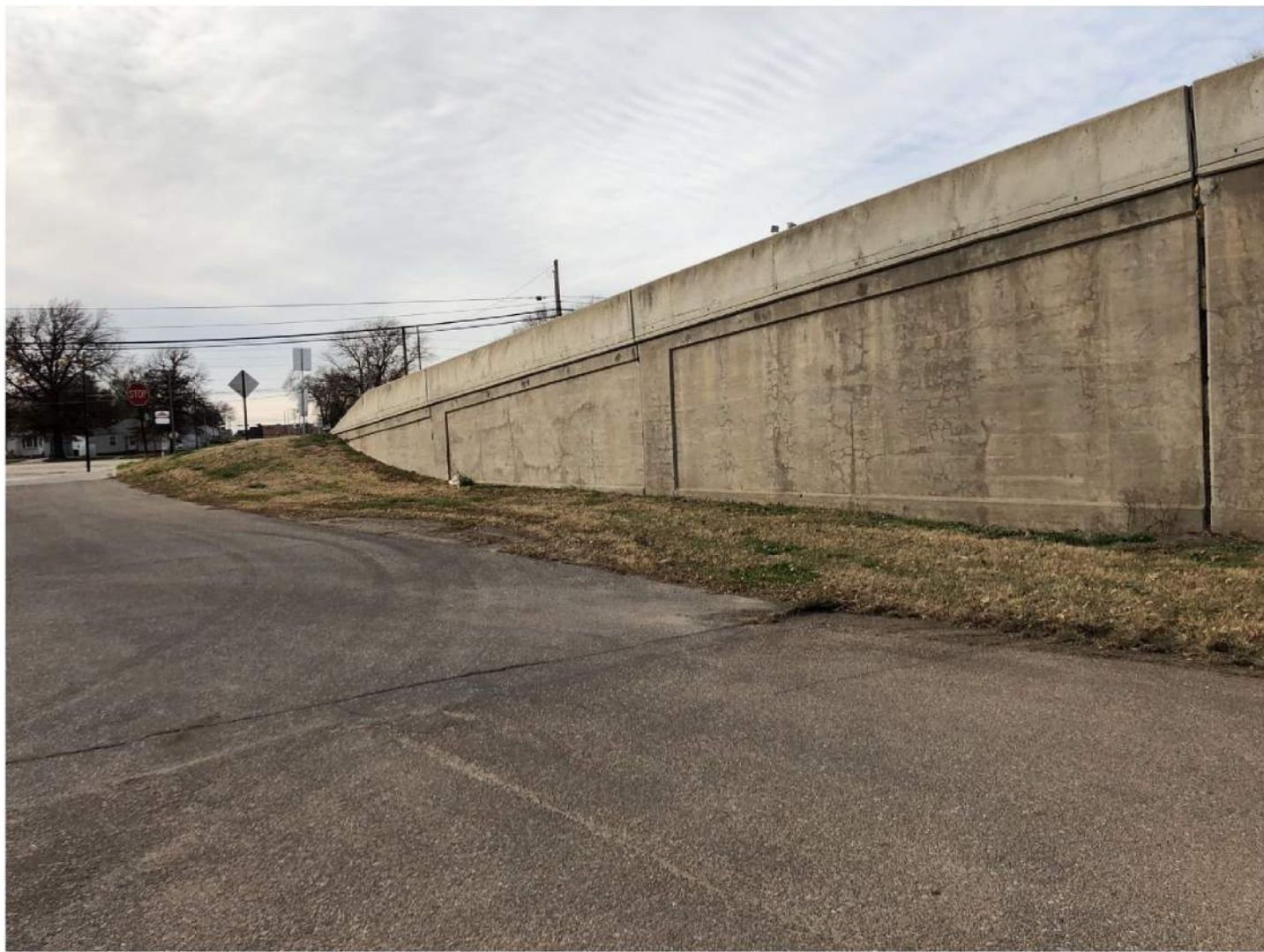
PHOTO 9 - WEST APPROACH RETAINING WALL SOUTH SIDE LOOKING WEST
