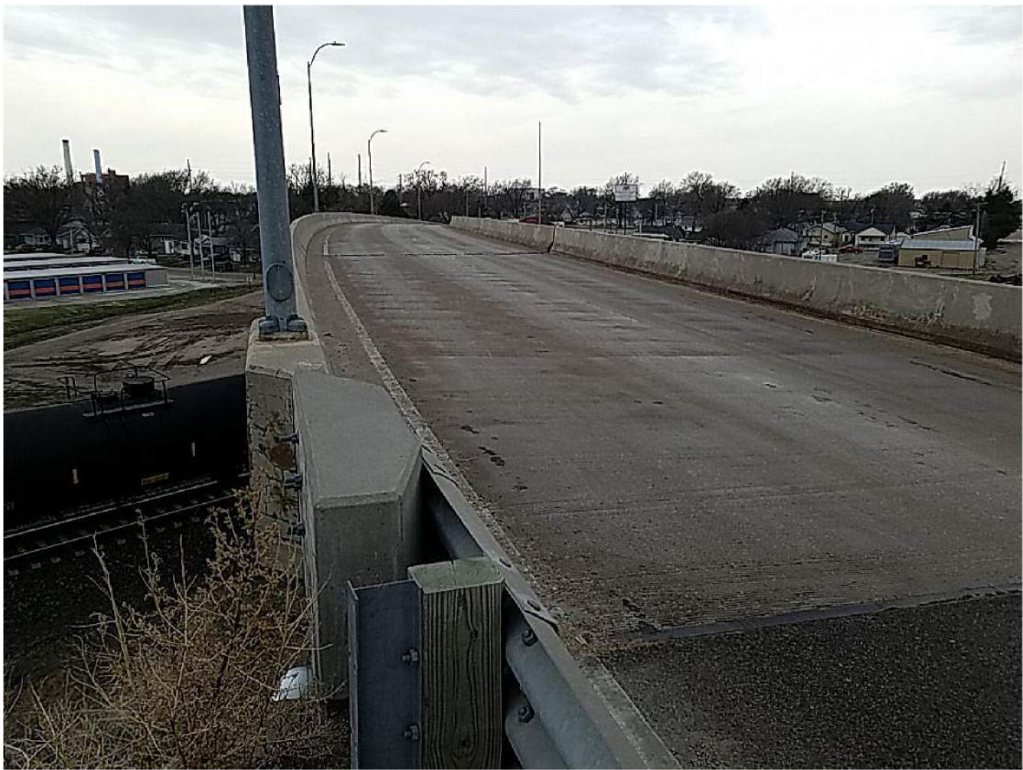
PHOTO 6 - LOOKING WEST AT DECK FROM ABUTMENT NO. 2
