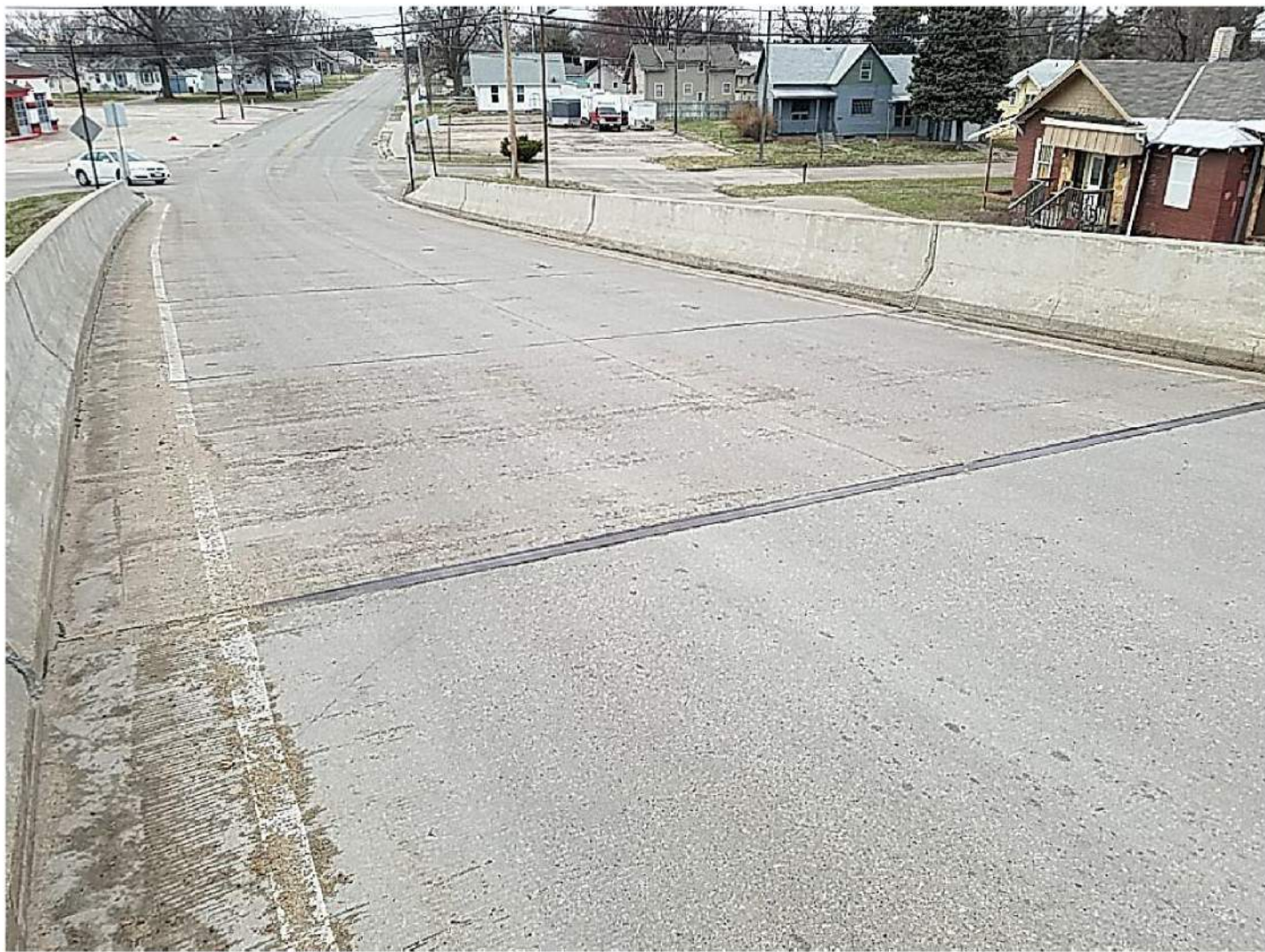
PHOTO 5 - LOOKING AT WEST APPROACH FROM ABUTMENT NO. 1
