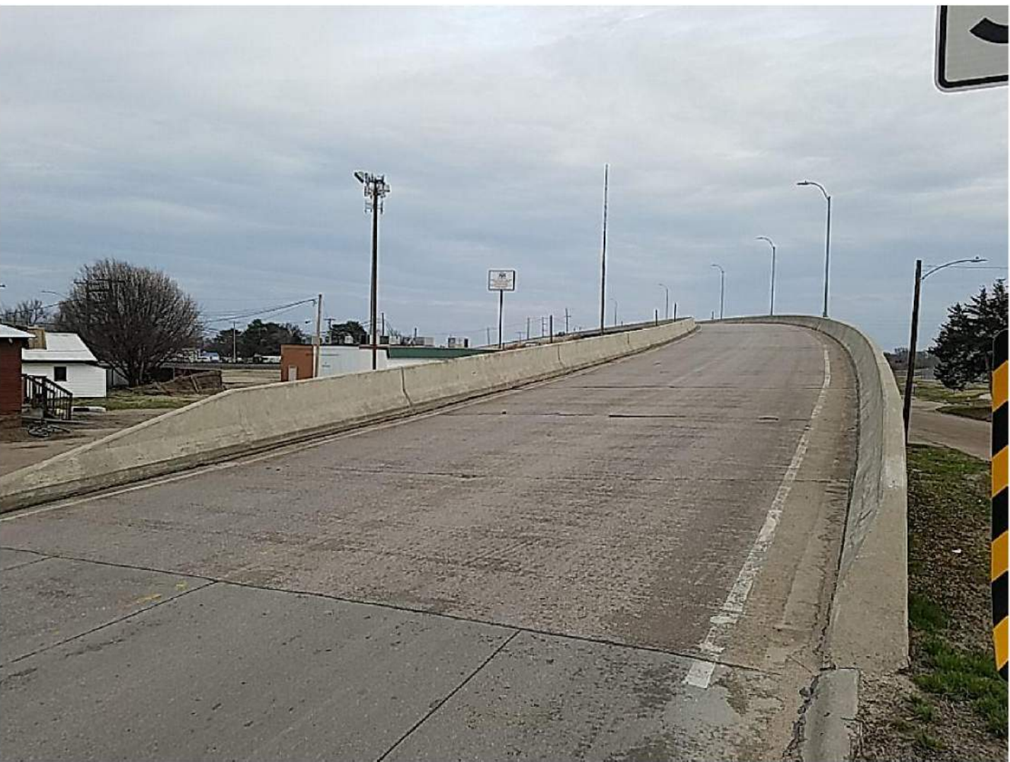
PHOTO 4 - LOOKING EAST AT DECK FROM WEST END OF WEST APPROACH RETAINING WALL
