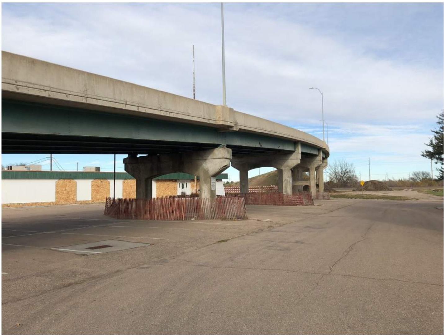
PHOTO 2 - LOOKING EAST ALONG SOUTH SIDE FROM ABUTMENT NO. 1
