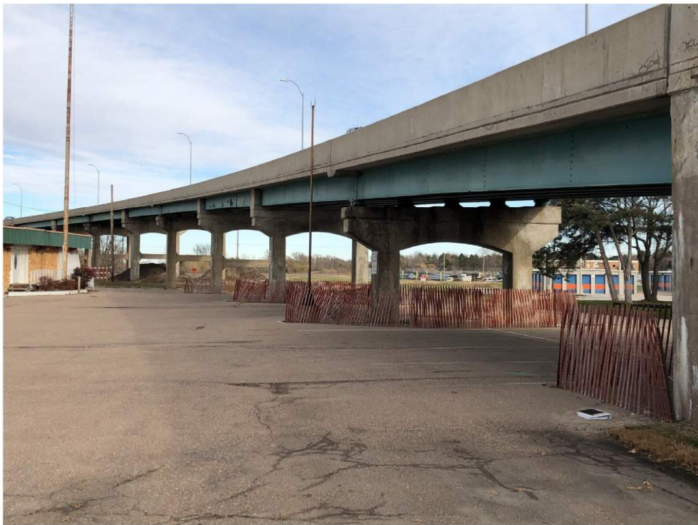
PHOTO 1 - LOOKING EAST ALONG NORTH SIDE FROM ABUTMENT NO. 1
