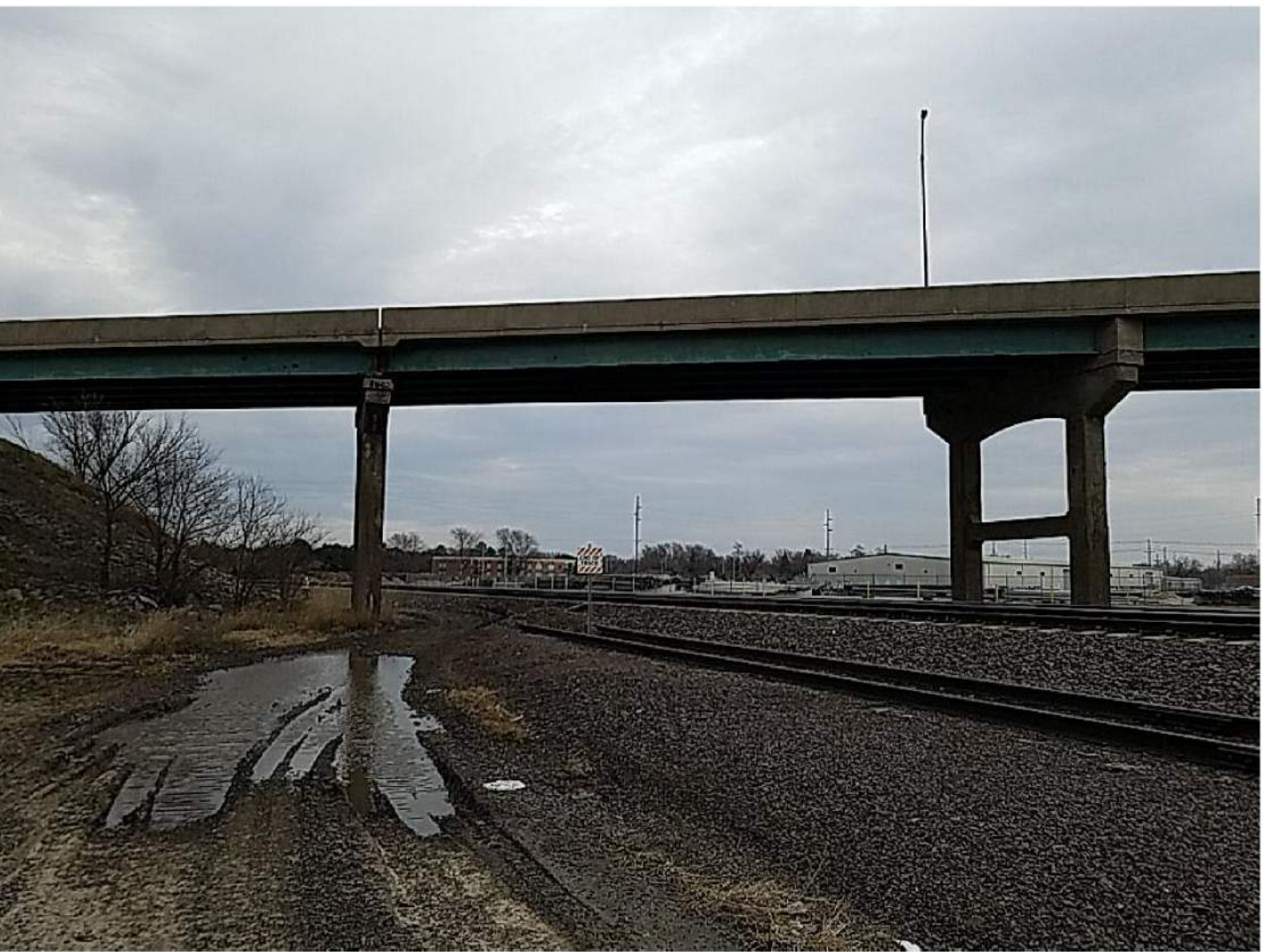
PHOTO 8 - LOOKING SOUTH AT UPRR TRACKS BELOW SPAN NO. 8
