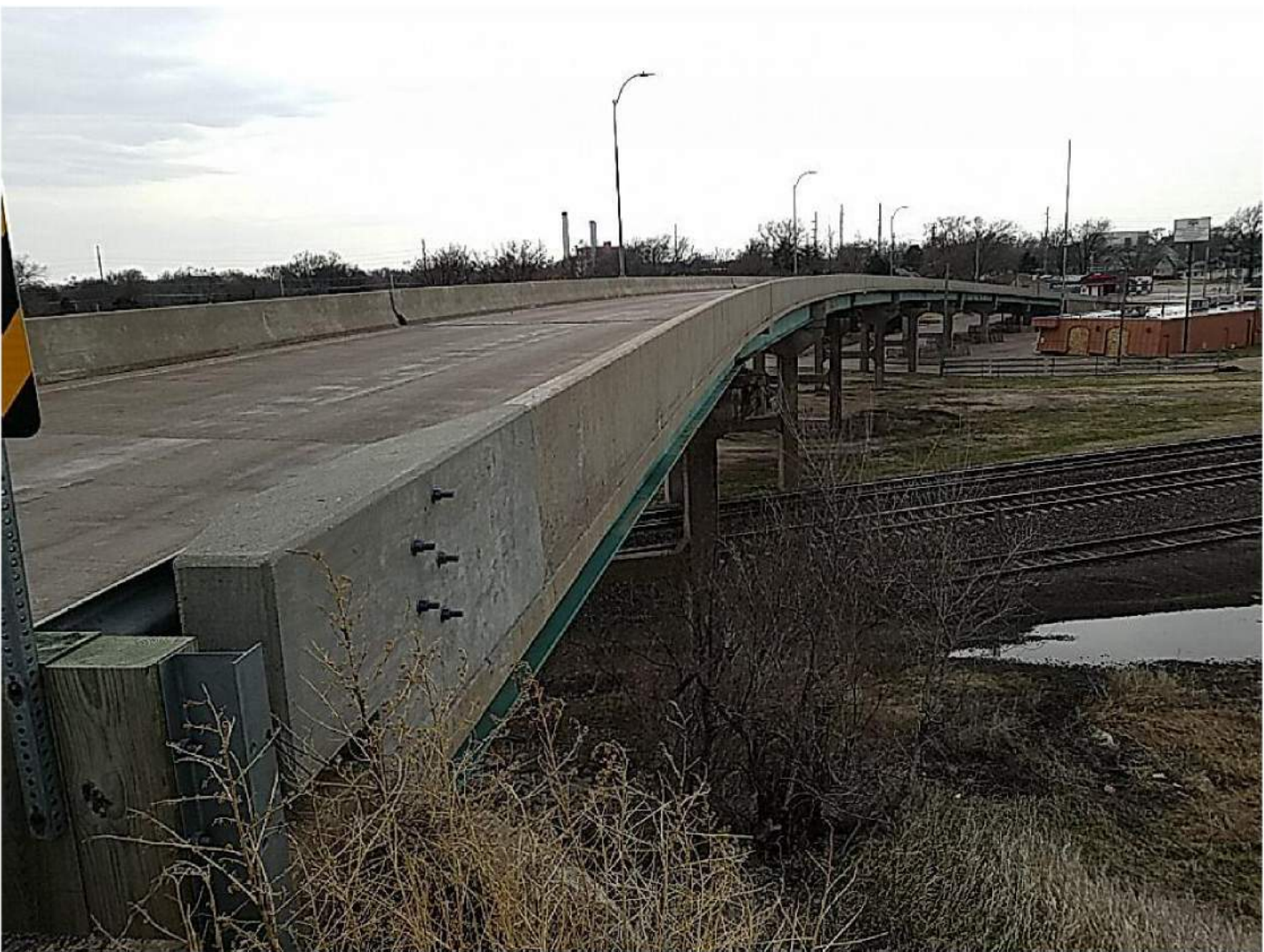
PHOTO 3 - LOOKING WEST ALONG NORTH SIDE FROM ABUTMENT NO. 2
