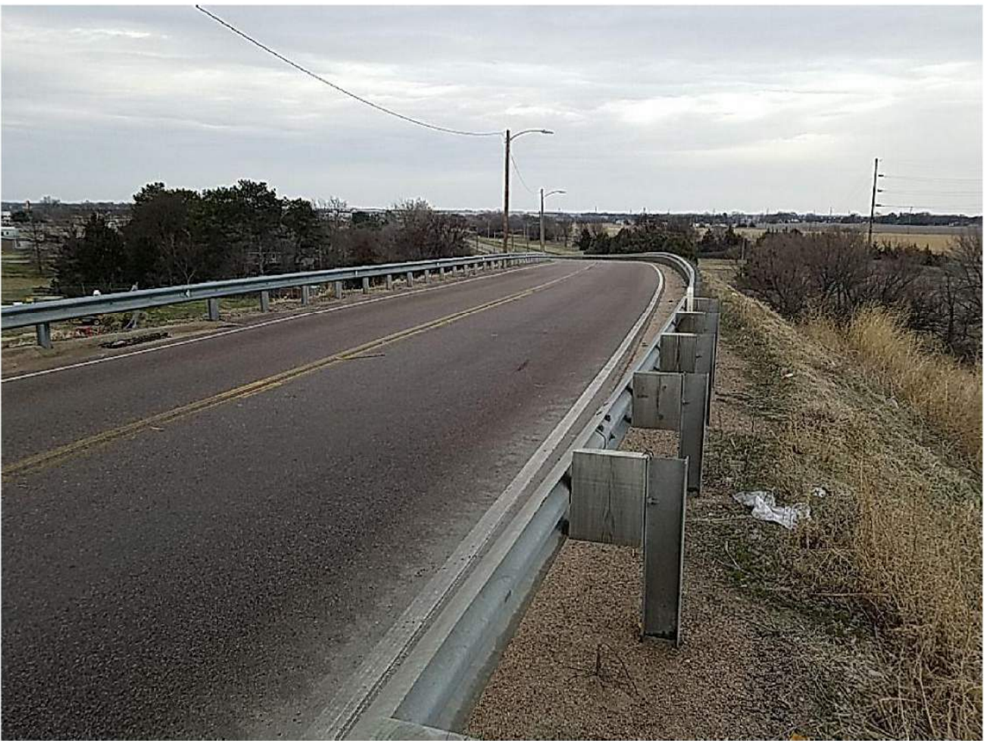
PHOTO 7 - LOOKING AT EAST APPROACH FROM ABUTMENT NO. 2
