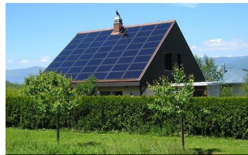
Example of a Solar Conversion System, Structure-mounted
