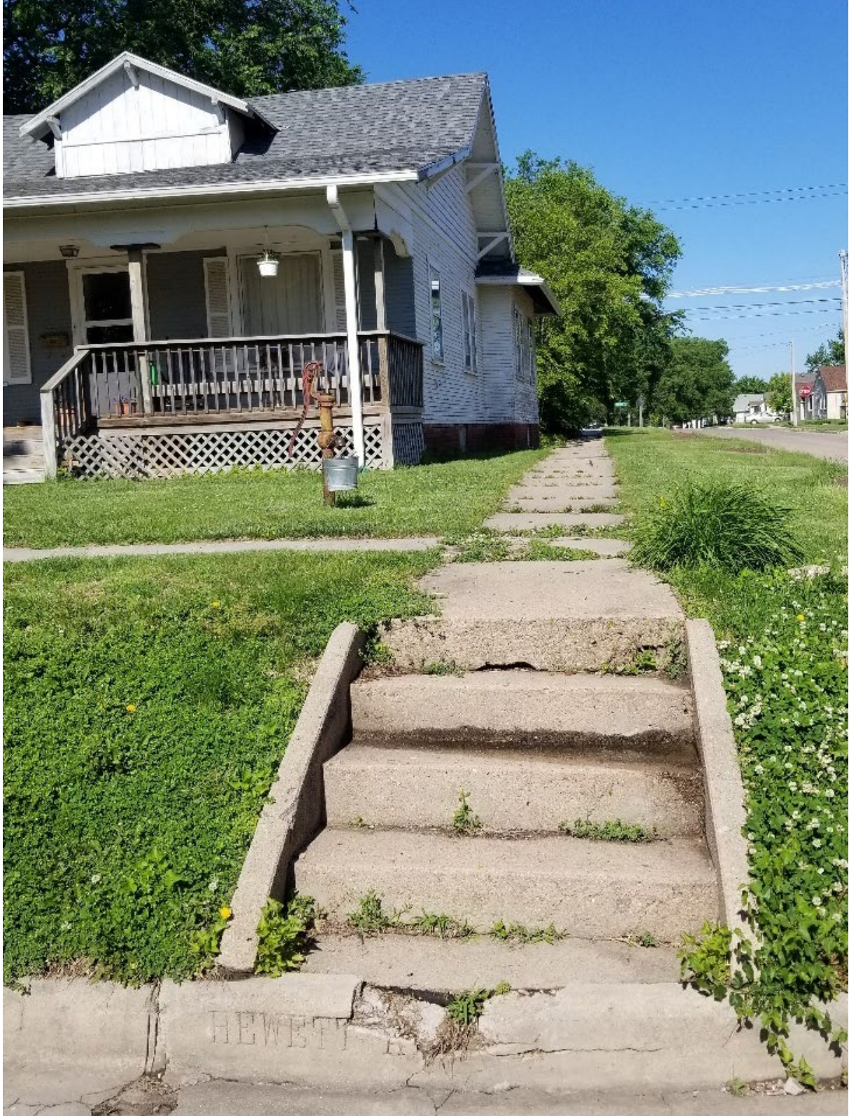
Figure 1.10 Stairs within the sidewalk
