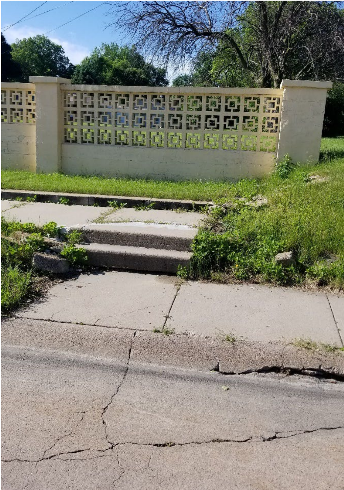
Figure 1.11 Stairs within the sidewalk
