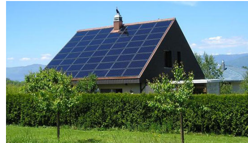
Example of a Solar Conversion System, Structure-mounted
