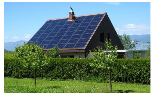
Example of a Solar Conversion System, Structure-mounted
