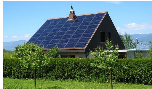
Example of a Solar Conversion System, Structure-mounted
